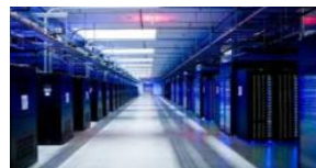
Data Center Renovation 100 MB
